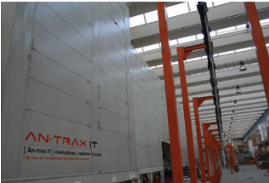
1 - Partial view of the paint plant installed at Antrax.
