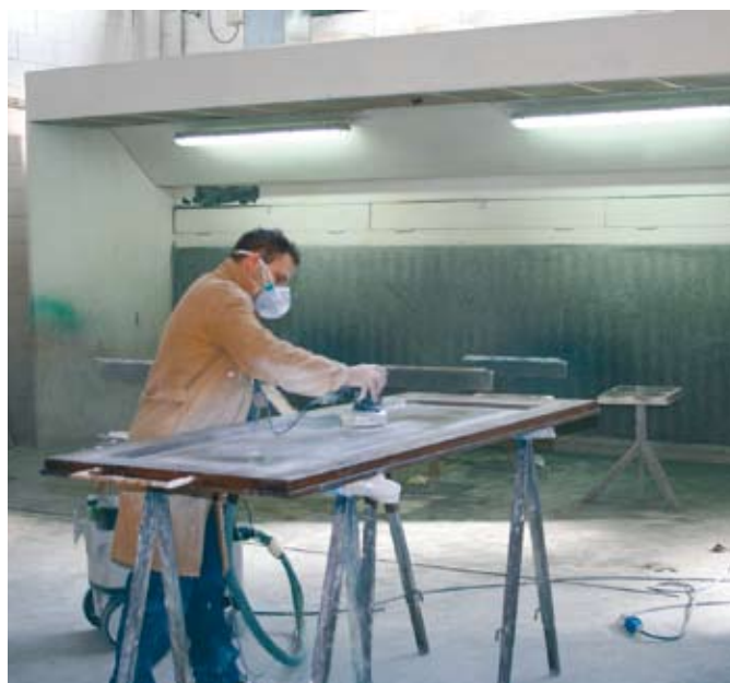
7 – The manual application in a dry booth, in the Monzio workshop.
